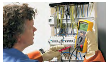
Insulation test at a distribution panel
